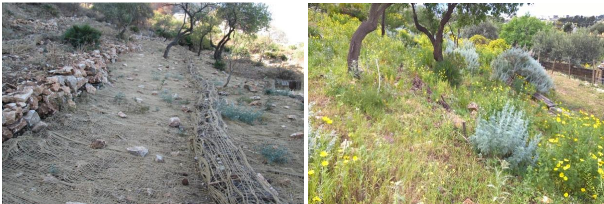
Fig.8 Slope Protection Biomat & Organic Pillows (Before in 2014 and after in 2017)
