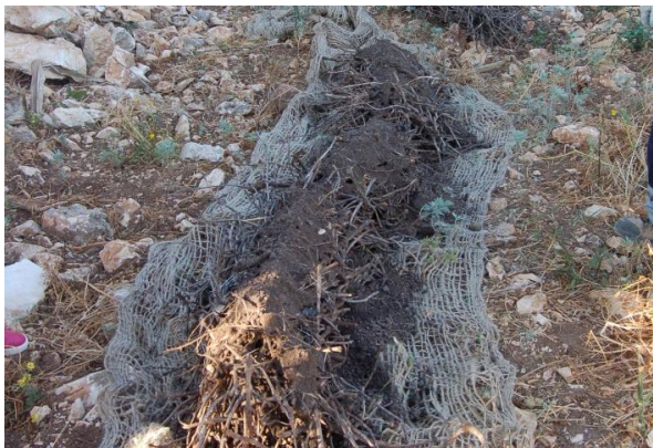
Fig. 6 Realization of bio-rollers with technosoils and vines pruning
