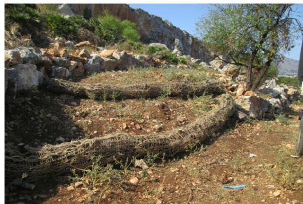
Fig. 6 Realization of bio-rollers with technosoils and vines pruning
